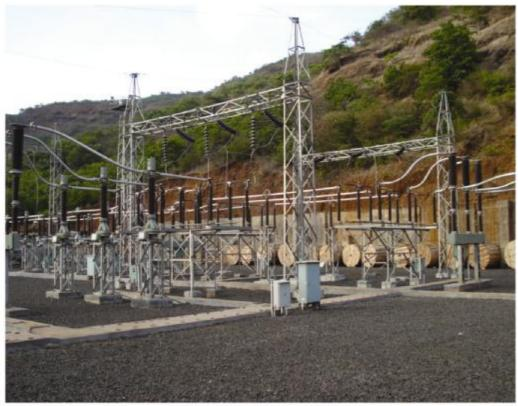
2x 25 MVA, 110 KV Switch Yard, Sub Station At Lavasa
